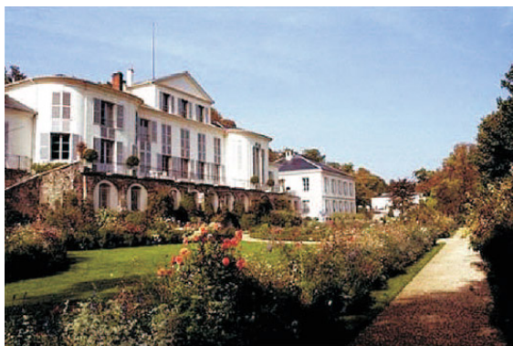
Figur 1. BIPM's hovedbygning, Pavillon de Breteuil. [1]
